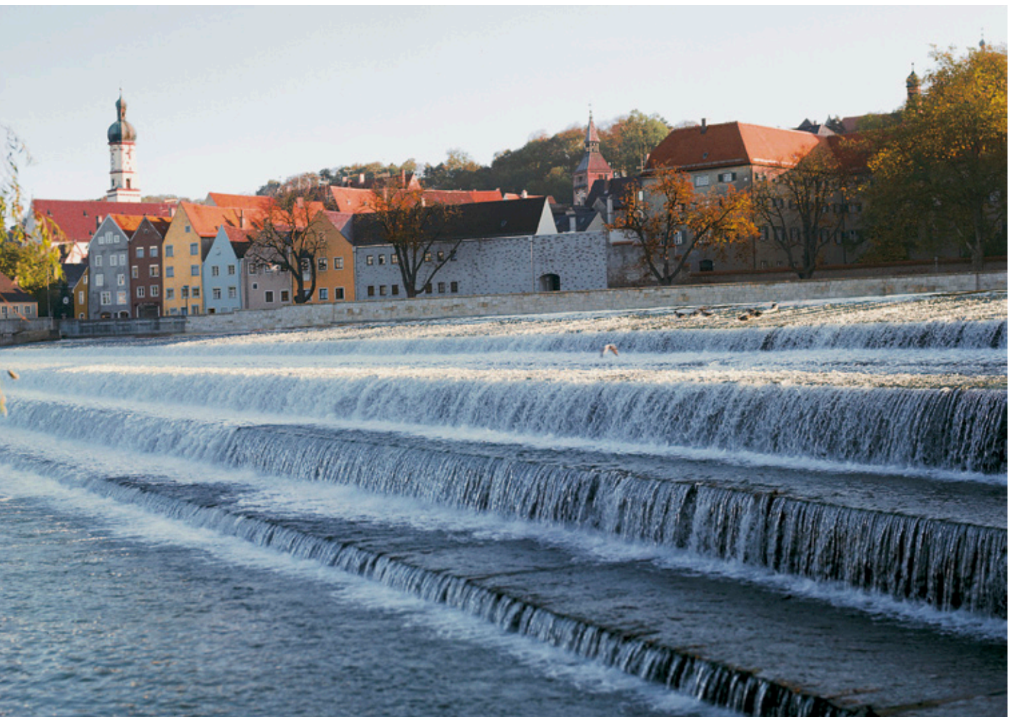
Das Lech-Wehr in Landsberg (Foto: © W. Binder LfU)
